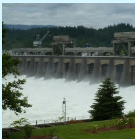
Bonneville Lock and Dam
