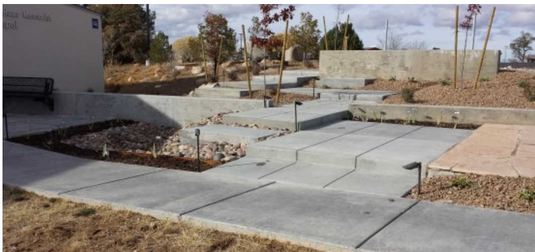
Embry Riddle University Memorial Garden site before construction (above) and after with partial planting (below).
